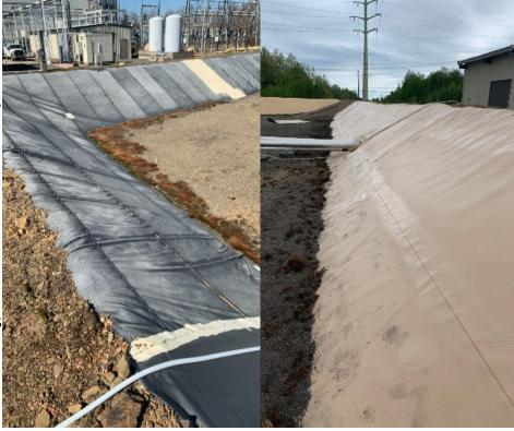
process of binding our polyurea liner to virtually any existing liner allows for us to repair any situation which arises in secondary containment fields. We trenched the top of the berm to secure the liner from wind uplift and tied into each corner. NEP Hazelton now has a berm covering which will last for years to come. Our unique process creates a monolithic liner system which comes with a ten year warranty.
